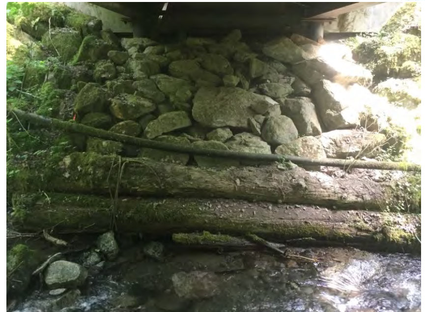
Left Bank Abutment when facing downstream
