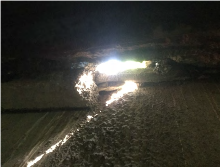
Damage to panel 1 at left approach
