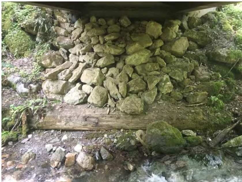
Right Bank Abutment when facing downstream
